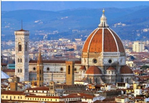
Dome of the Florence Cathedral Filippo Brunelleschi
